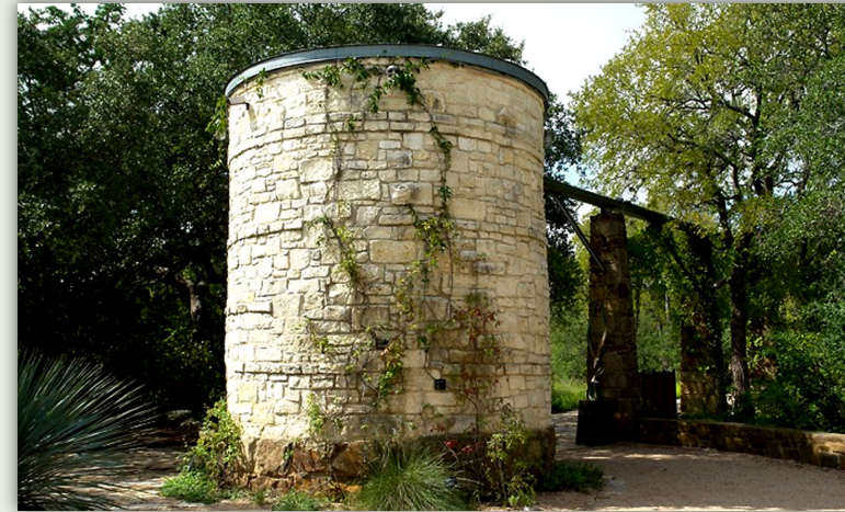
Rain water is captured and stored in this cistern, and used for landscape irrigation. (Lady Bird Johnson Wildflower Center, Austin, TX)
