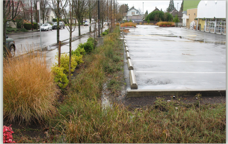
Vegetated swales clean storm water runoff from parking lots and allow it to infiltrate the earth.
